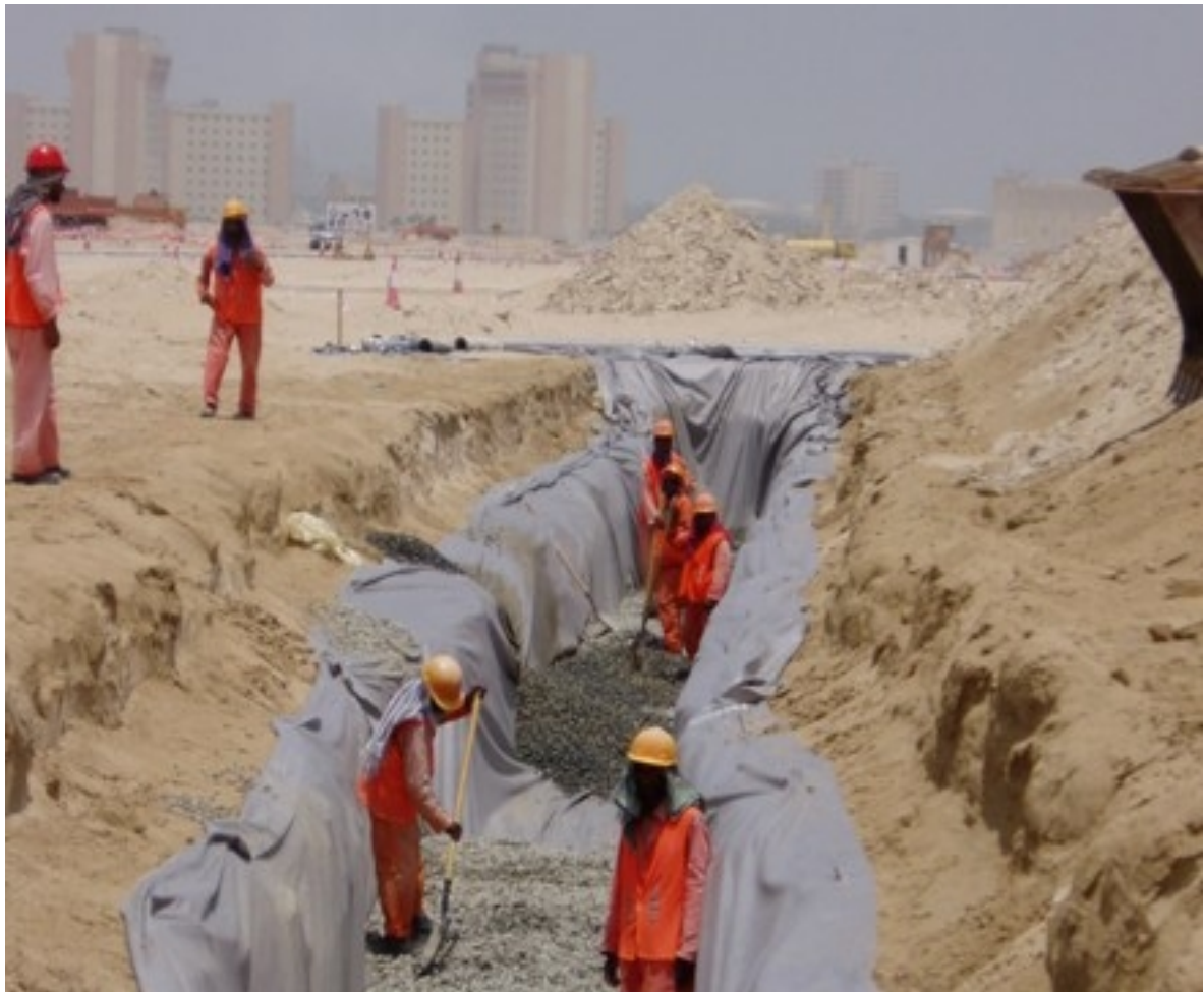
Construction Workers on Site
