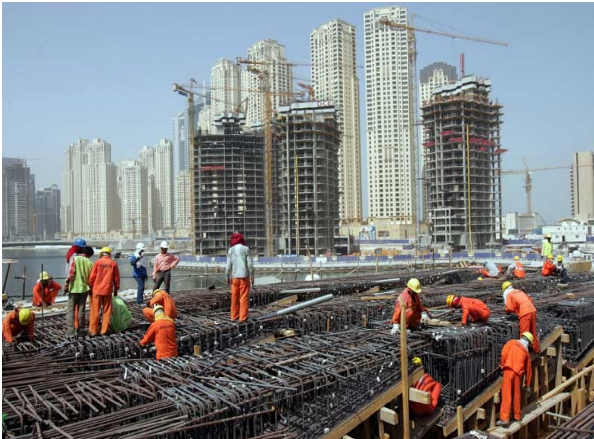
Workers in a construction site
